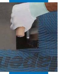
Waterproofing with Mapelastic reinforced with Mapenet 15<u>0</u>
